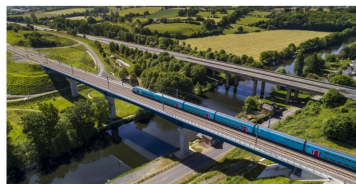
High Speed Line Bretagne-Pays de la Loire, France
