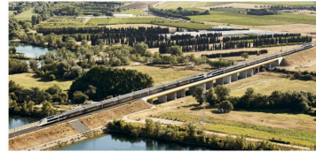
High Speed Line Nîmes-Montpellier (CNM), France
